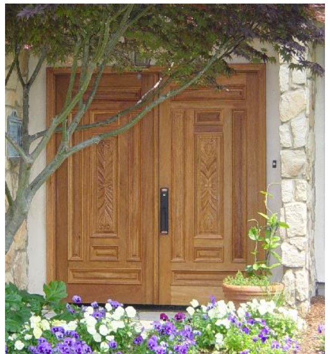
#1203-CP Doors Installed as Courtyard Doors
